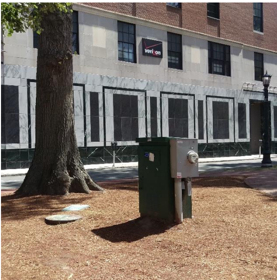
Box on Worthington/Stearns Square Dimensions: 28" x 14" x 45"h One side obstructed by 19x22" utility panel.
